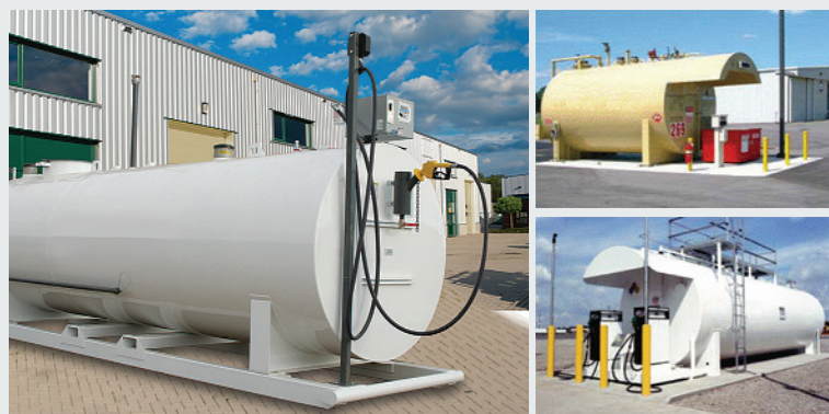
In 2010, all gasoline-dispensing facilities in California that featured ASTs for product storage needed to be compliant with CARB's certification procedure for Enhanced Vapor Recovery.
